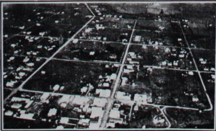
This unique photograph of part of the residential area of Opotiki, and showing a few of the business premises, was taken from an aeroplane. It clearly demonstrates the care that was taken in laying the town out. Photo, G. S. Shalloon.
